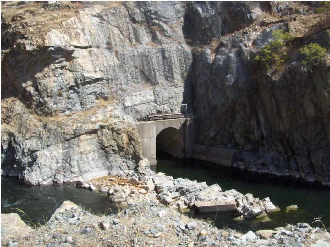
Figure 2.4-2. Don Pedro Dam - low level outlet works tunnel discharge.
