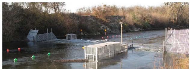
Figure 5.3.2-3 Fish counting weir at RM 24 on the lower Tuolumne River.
