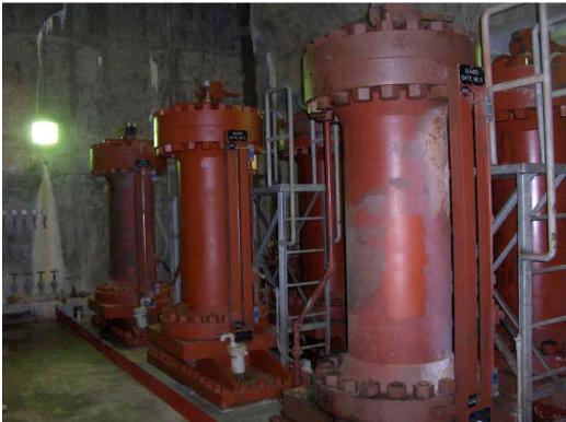
Figure 3.4.3-1 Don Pedro Dam - gate operators for the low-level outlet works.
