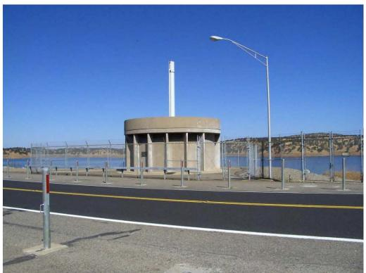
Figure 3.4.4-1Don Pedro Dam - power tunnel gate housing.
