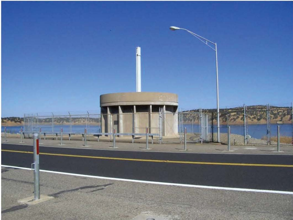
Figure 2.5-1. Don Pedro Dam - power tunnel shaft and gate housing.
