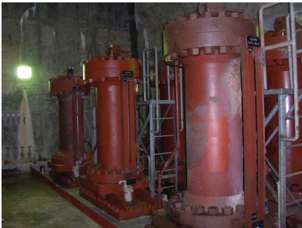
Figure 2.4-1. Don Pedro Dam - gate operators for the low level outlet works slide gates.
