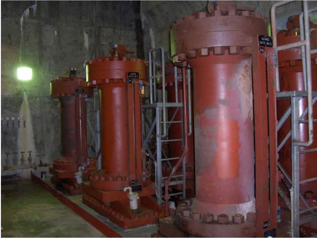
Figure 2.1-3. Don Pedro Dam - gate operators for the low level outlet works slide gates.
