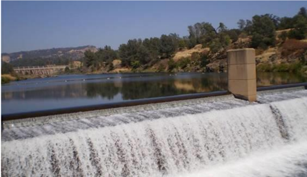
Figure 2.2-2. Photograph of the fish barrier weir installed on the Feather River, below Oroville Dam. The fish counting and barrier weir proposed for the Tuolumne River will be a similar type of barrier weir.
