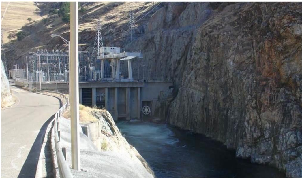
Figure 2.1-6. Don Pedro powerhouse and hollow jet valve viewed from tailwater.
