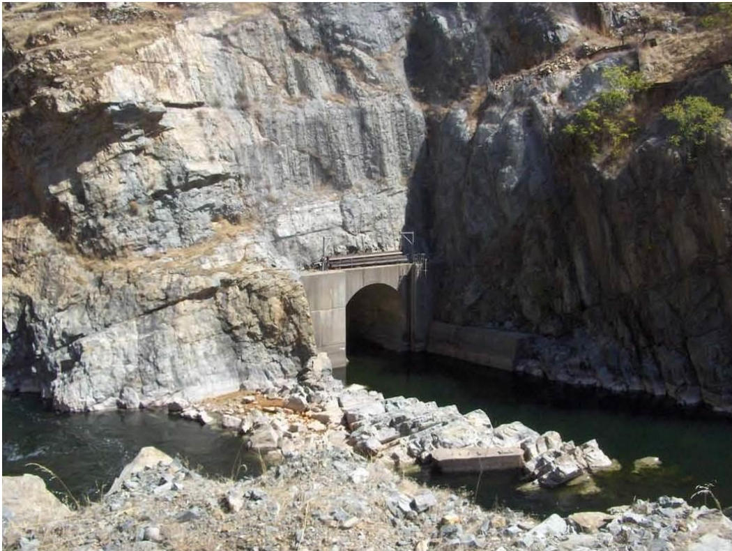
Figure 2.1-4. Don Pedro Dam - low level outlet works tunnel discharge.
