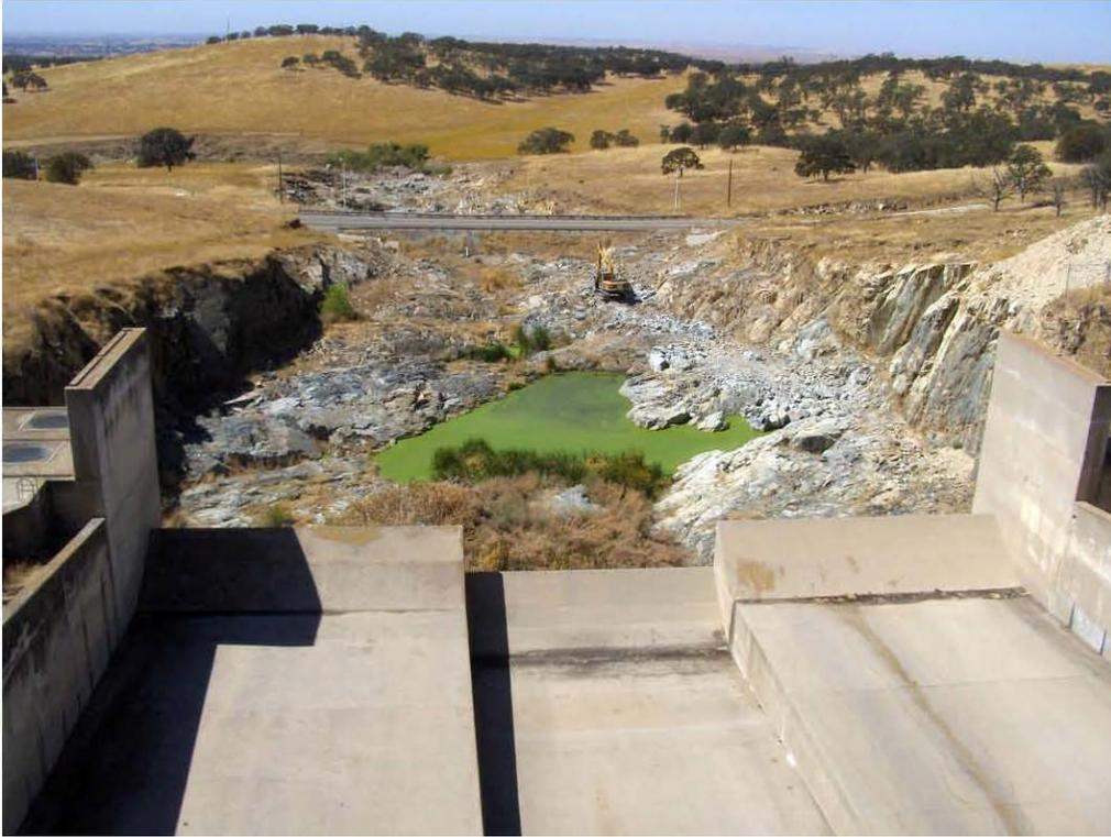
**Figure 3.4.2-2 Don Pedro spillway discharge channel.**
