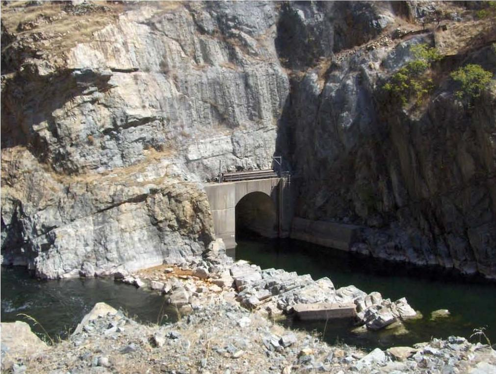
**Figure 3.4.3-2 Don Pedro Dam - downstream exit from outlet works tunnel.**
